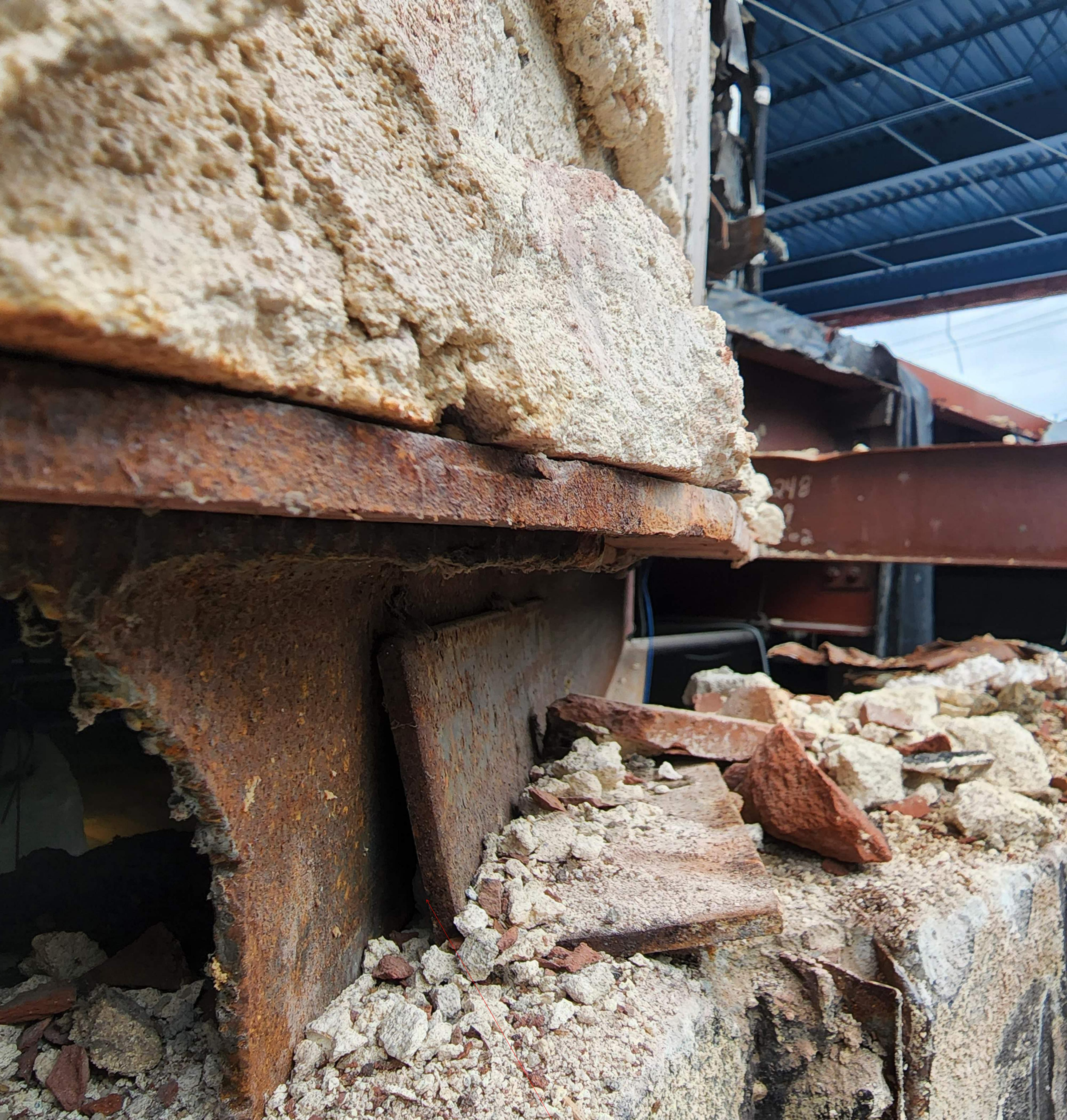
EXISTING BEAM IS COPED AND IMPROPERLY SUPPORTED
