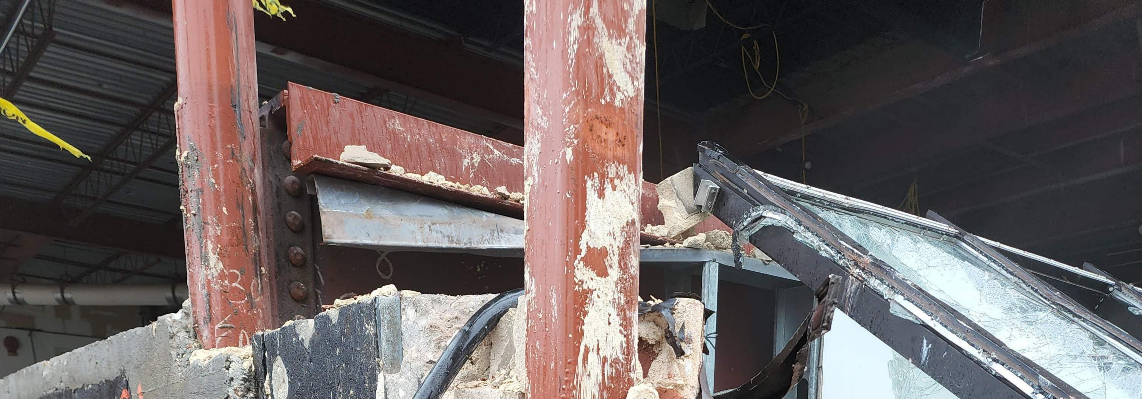
COLUMN APPEARS TO EXTEND FURTHER DOWN INTO BRICK PIER BUT COULD NOT CONFIRM.
