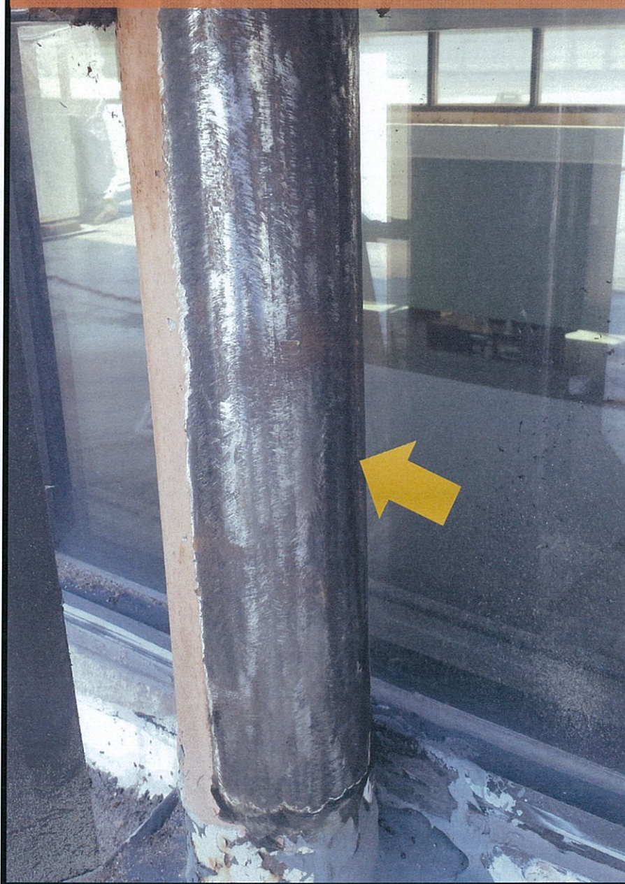
1. LINTEL WORK (PREPARATION + PROGRESS)
