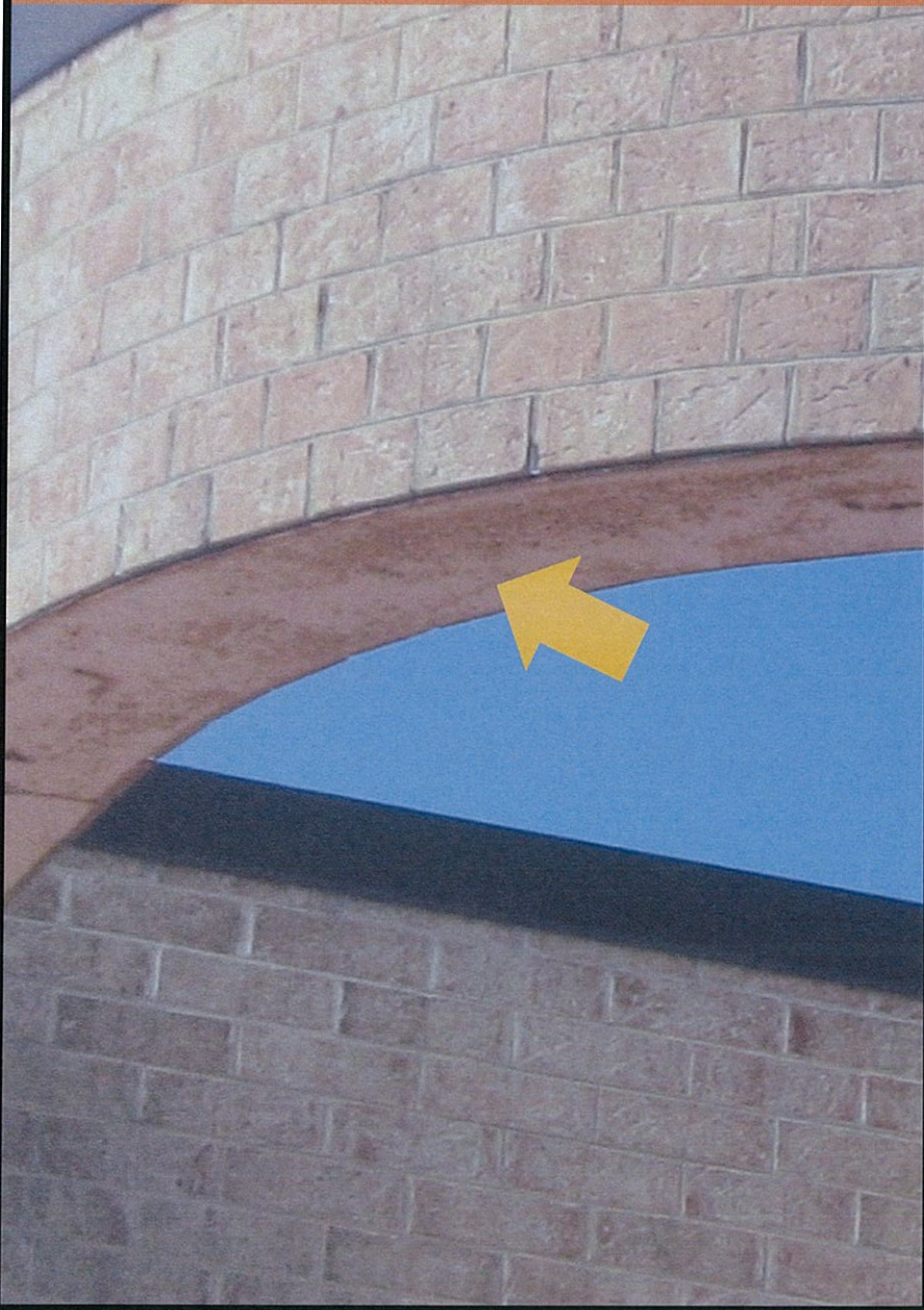
1. LINTEL WORK (BEFORE)
