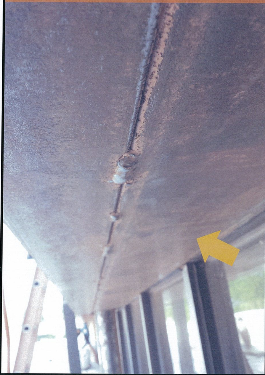
1. LINTEL WORK (PREPARATION + PROGRESS)
