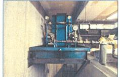
BECAUSE OF BOTH THE BOILER'S AGE AND THE INEFFICIENCY CREATED BY USING STEAM TO HEAT WATER, THE BOILER SHOULD BE CONSIDERED FOR REPLACEMENT WITH ROOF TOP UNITS SIMILAR TO THOSE IN SERVICE ON THE 1982 SECTION.
