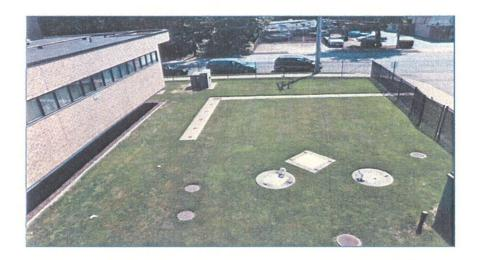
BASED ON CONVERSATIONS WITH MAINTENANCE PERSONNEL AND GENERAL INFORMATION ABOUT THESE SYSTEMS, IT DOES NOT APPEAR THAT IT IS OPERATING CORRECTLY. THE RESULT IS THE DISCHARGE OF AN EXCESS OF NITRATES IN TO THE GROUND AND EVENTUALLY THE WATER TABLE.
