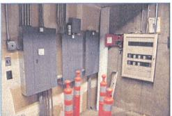
THE MAIN DISCONNECT SWITCH IS 1600 AMP AND WITH 80% SAFETY FACTOR, THIS EQUALS APPROXIMATELY 1280 AMPS
