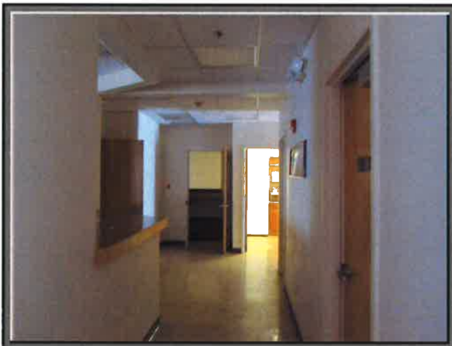
Interior - View Facing West
