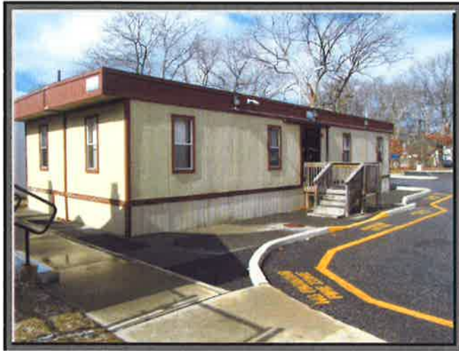
Fixed Trailer - Facing Northwest
