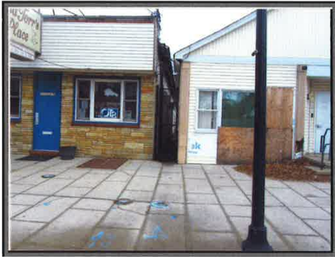
West Side of Building
