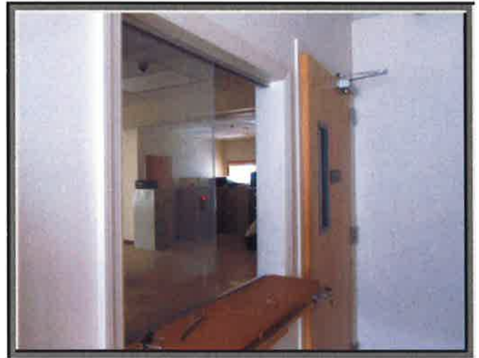
Rear Entrance - Foyer
