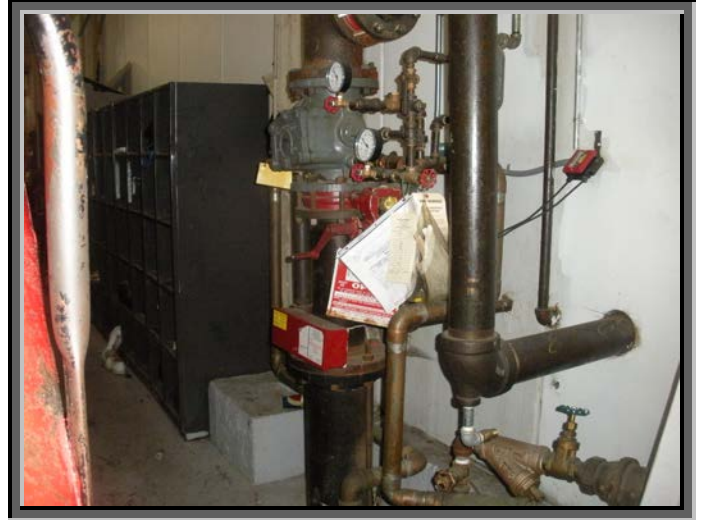
Fire Sprinkler Controls
