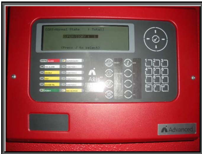
Alarm Control Panel
